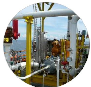
An FGR system is designed to capture waste gases that would go to the flare tip during normal operations. The FGR system is located upstream of the flare to capture and recover some or all of the waste gases before they are flared. Most flares operate at pressures just above atmospheric pressure, and therefore the gas must be compressed to a higher pressure for transport throughout the plant and for use at the intended destination.
